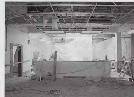
The old New Zealand Room in the City Gallery, Wellington under construction, 1993. Photo: Neil Price
